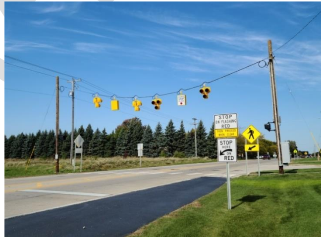
Figure 7: The photo above shows the new HAWK pedestrian crossing on Pine Road between Youngs Ditch Rd looking North to Ridge Road in Hampton Township. This is the very first HAWK signal used in Bay County.
